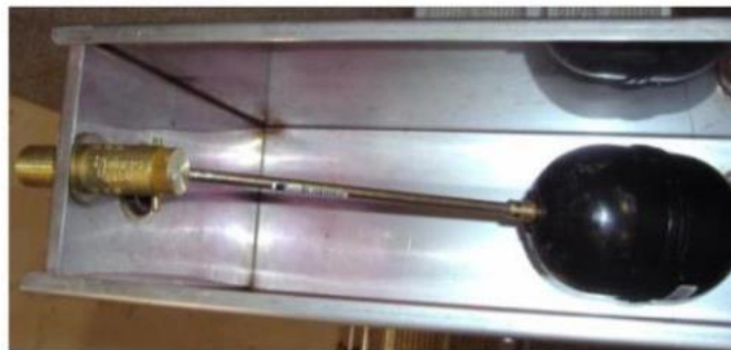
Top-up tank view from above
